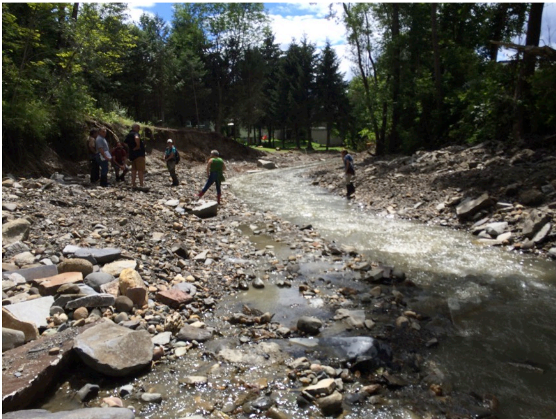
Left bank failed during July 2015 storm
